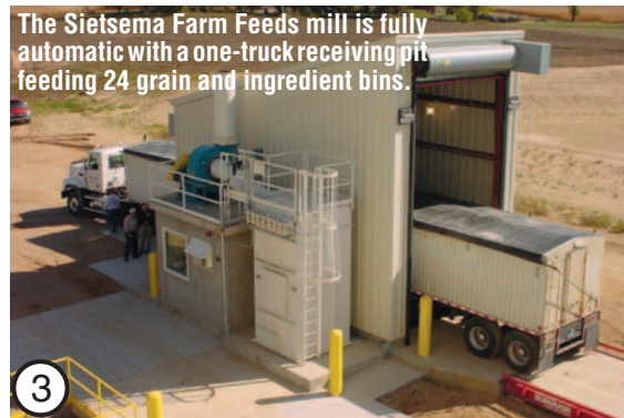
A four-ton weigher is capable of moving to three positions, being automatically filled and then moving to the truck hopper for discharge.
